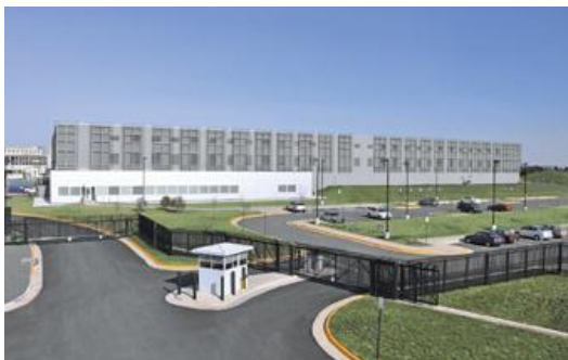
MTU Onsite Energy generator sets back up LEED-certified COPT DC-6 (formerly Power Loft I @ Innovation) Data Center.
