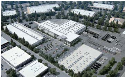
Vantage Data Centers' campus in Santa Clara, California, uses novel energy-saving techniques and emergency standby generator sets from MTU Onsite Energy for building V2.
