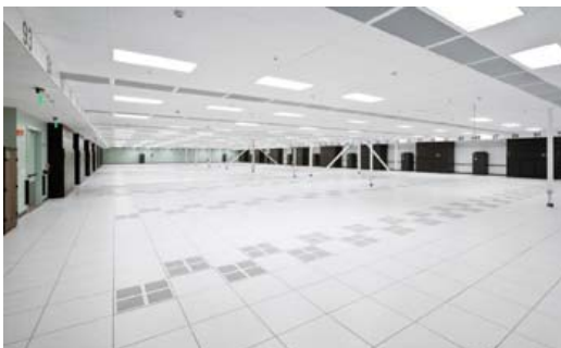
A photo of an empty server floor at one of Vantage's Santa Clara data center buildings, taken soon after construction and before tenant move-in.
