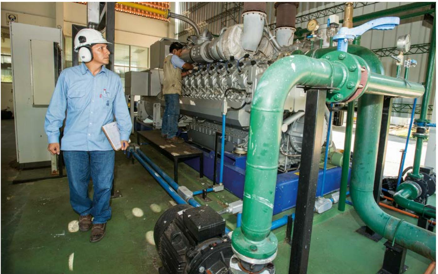
The digester is 23 feet deep with an area of 430 square feet and holds roughly 1.6 million gallons of biomass. The biomass is mixed and fermented to produce biogas with a methanol content of between 50 percent and 60 percent. Before the gas is pumped to the engine, it is passed via underground pipes through an active carbon filter that reduces the sulfur content.
