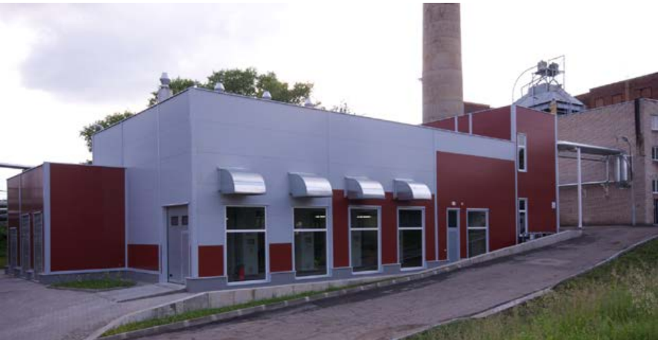
The new building for the CHP systems was constructed according to BMG's specifications. (Image: Baltic Marine Group)
