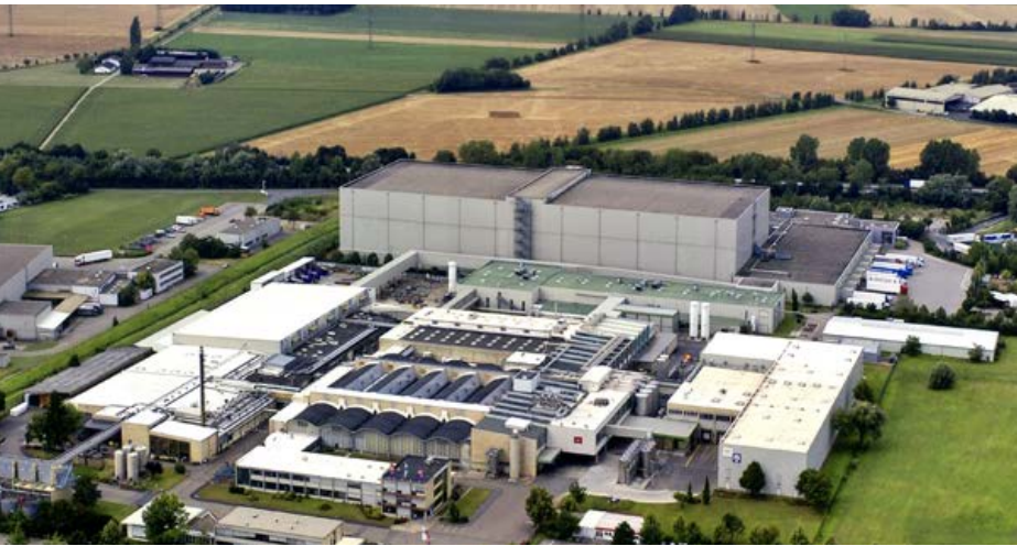
A Rolls-Royce cogeneration plant supplies heat and power for the Langnese ice cream factory. (Picture: Langnese Heppenheim / Unilever)
