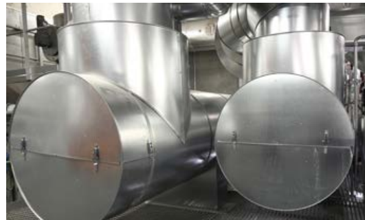
The low-temperature exhaust gas heat exchanger (right) boosts fuel efficiency by an additional three percent. (Picture: MTU/Ralf Dunker)
