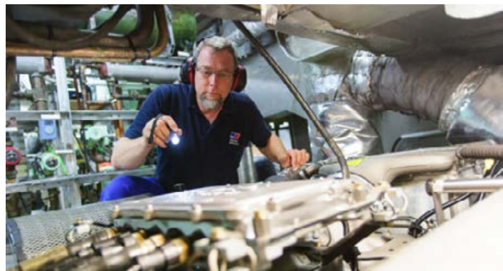
In the pilot launch Duhnen, two MTU Reman engines of type 12V 2000 M70, each generating 788 kW output, provide the right propulsion. Rolls-Royce Field Service Inspector Detlef Paul assesses the engines. They have a harsh life, with up to 6,000 operating hours a year. (Pictures: Rolls-Royce)
