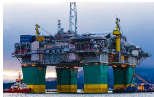
End of 2010, the Gjøa field off Norway’s west coast came on stream. The fire extinguisher pumps are driven by four MTU 20-cylinder Series 4000 engines. (Picture: Tommy Solstad)
